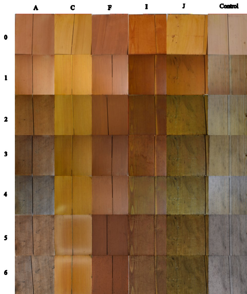
Figure 4.3 Visual changes of uncoated and coated CLT samples after 6 months of natural weathering in Starkville, MS
